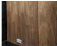
STAINED PLY FINISH WITH SHADOWLINES
